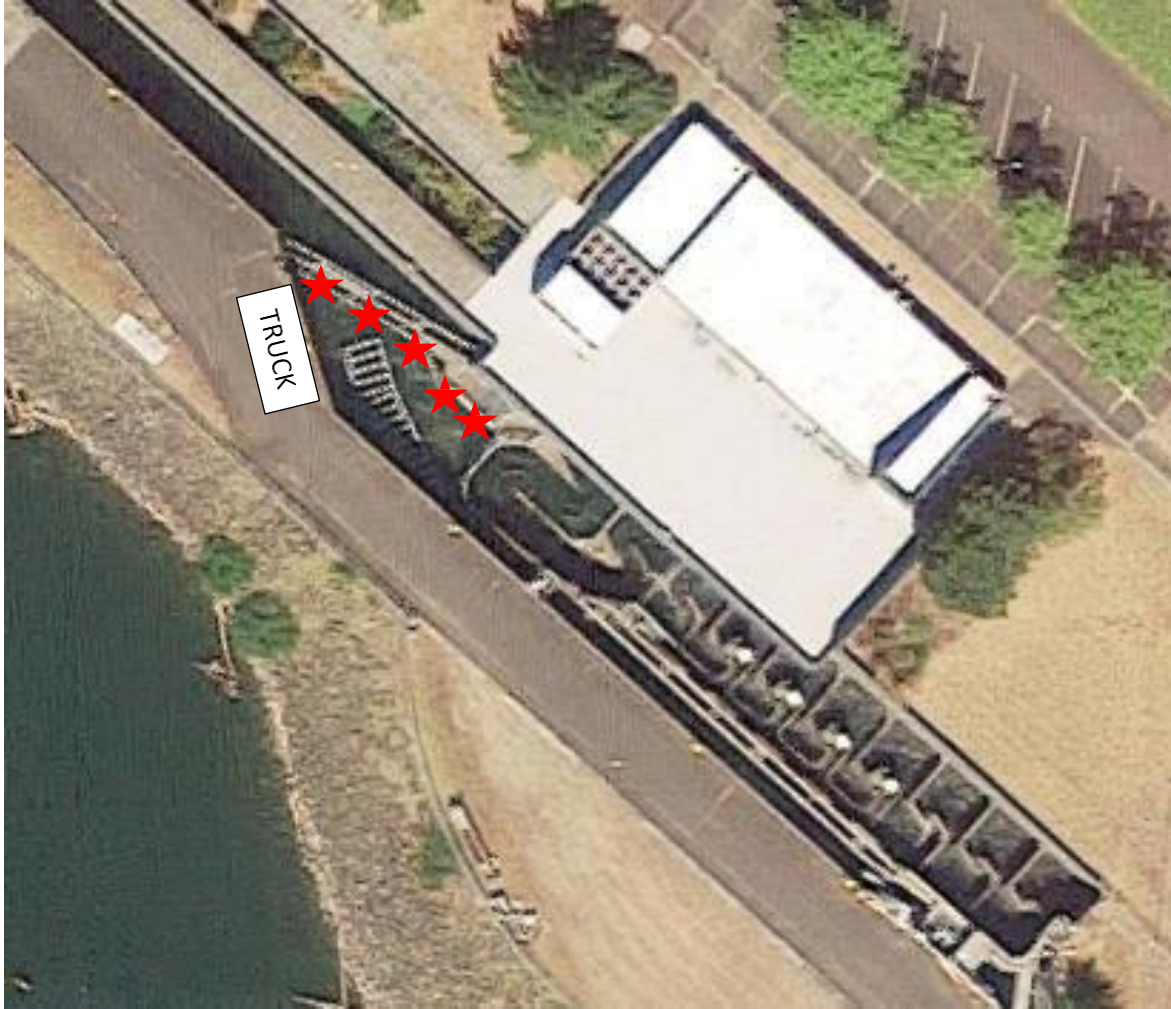
Figure 4. Close-up aerial view of the Bonneville Dam Washington Shore Fish Ladder at the count station and visitors center. Potential trap locations above picketed leads are denoted by red stars. Alternate locations may be selected upon consultation between USACE and CRITFC member Tribes.
