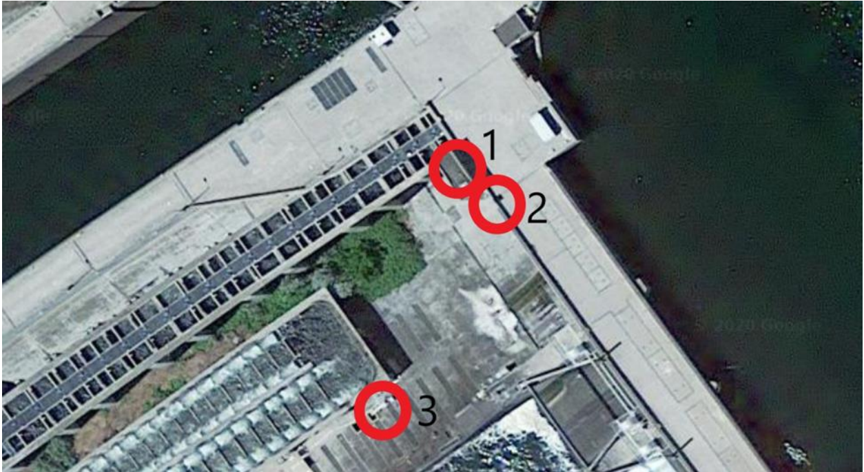
Figure 12. Close-up aerial view of the JDA North Fish Ladder showing the location of the JDA North lamprey flume trap rest box on the deck of the dam (3). Red circles 1 and 2 show the location of the elevator and the davit arm that can be used to lift buckets when elevator is inoperable.
